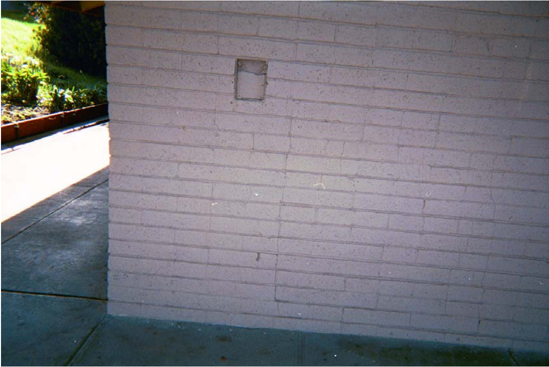
Figure 16: Vertical Cracks in CMU Walls
