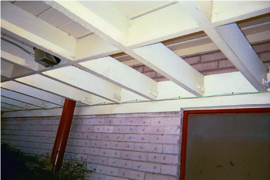
Figure 15: Holes in CMU Walls
