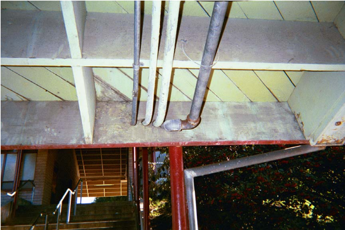
Figure 17: Pipes and Conduit at Covered Walkways
