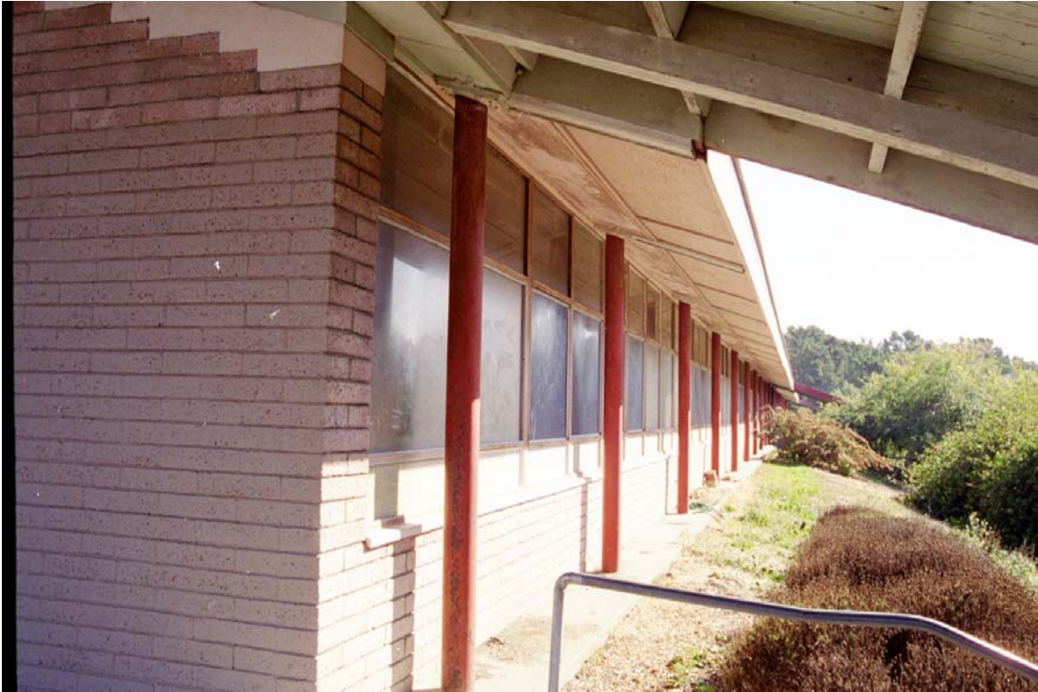
Figure 8: Rear Wall of Classroom Building
