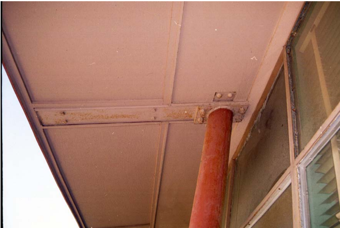
Figure 4: Rusting Steel at Overhangs
