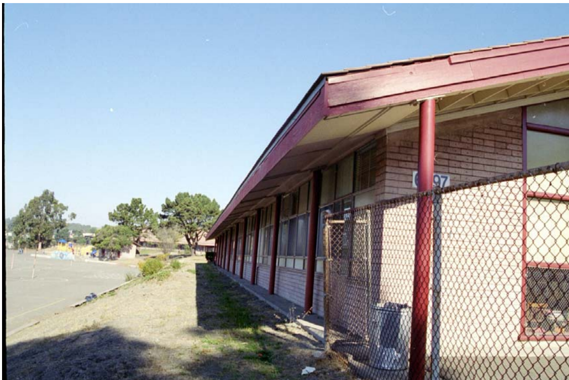
Figure 11: Rear Wall of Kindergarten Classrooms
