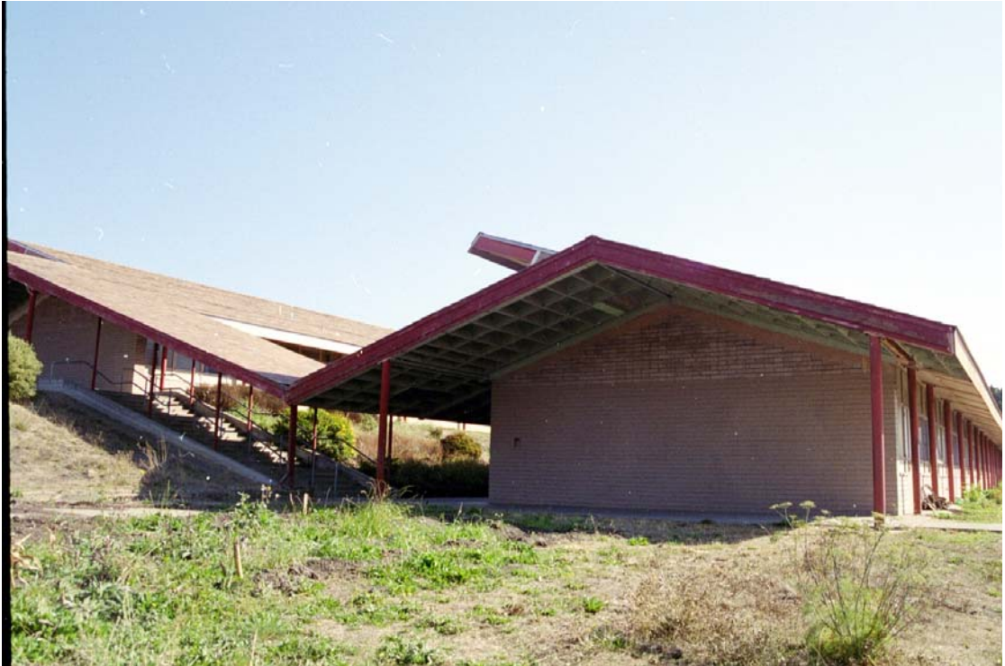
Figure 9: West View Classroom Buildings
