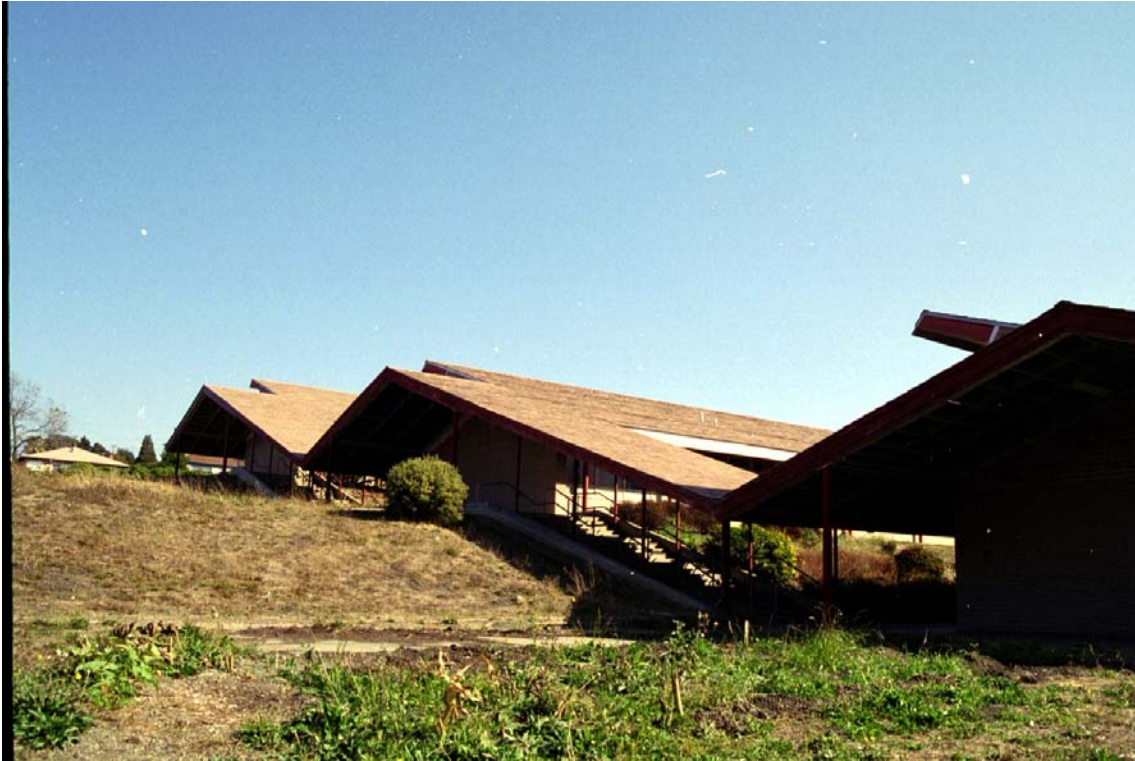
Figure 3: Covered Walkways Between Buildings
