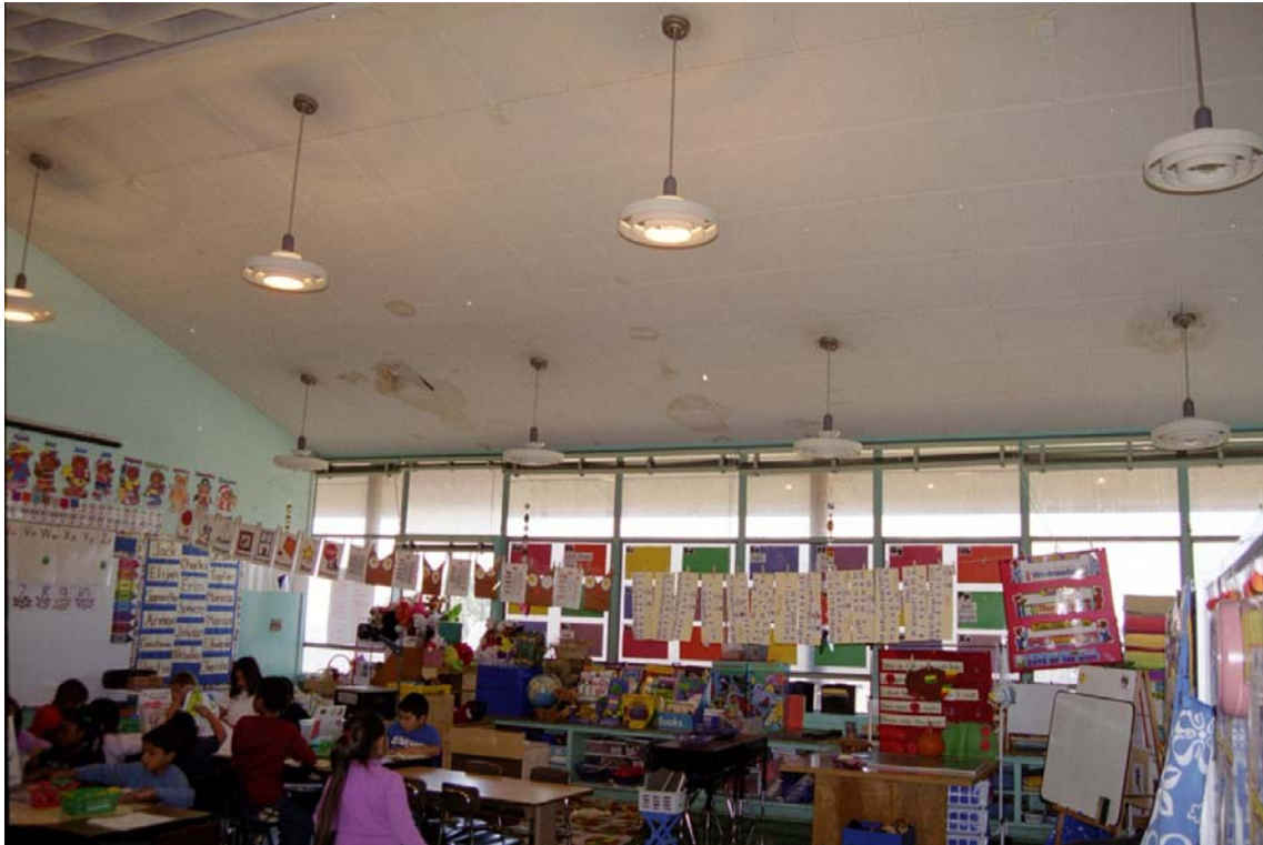
Figure 7: Water Stains on Classroom Ceilings
